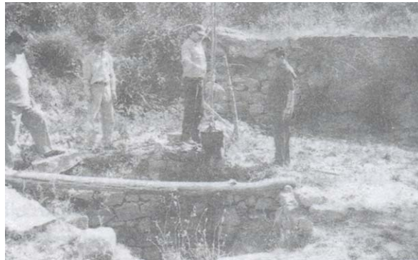
Fig.8 : Dungali at Koke-Baggi with load & bucket arrangement to lift the water (The depth of water is 1.8 meters from the surface)
