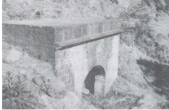
Fig.4 : Prolonged neglect has taken its toll and the bawari at Ghadda lies silted up
